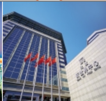
Beijing New World Centre Phase I
